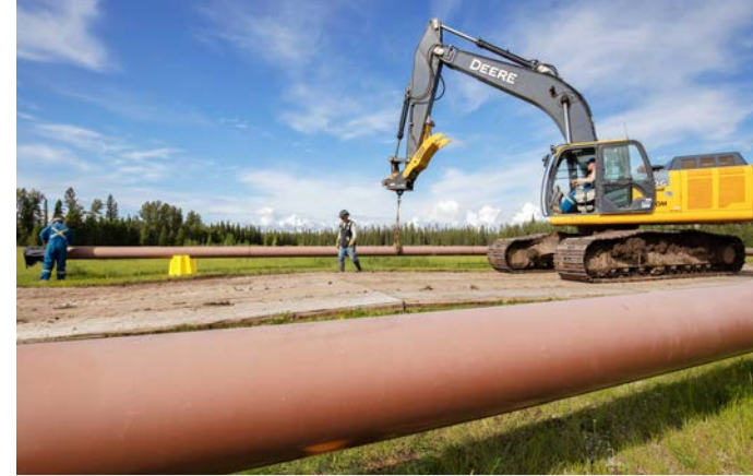
PMC crews preparing pipe for HDD
